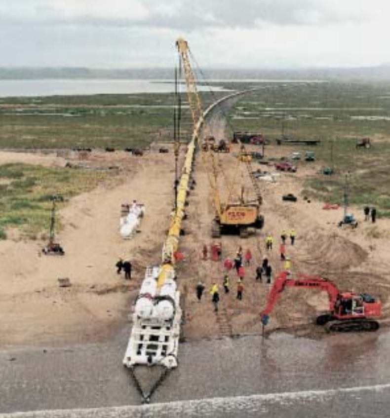
The launch of the Elgin/Franklin interfield pipeline bundle in Tain, 16 May 1999.
