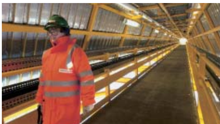
Crossing the bridge from the Elgin wellhead platform to the Elgin PUQ. As well as giving access for personnel, this 90-metre structure provides a route for process pipework and utilities.
