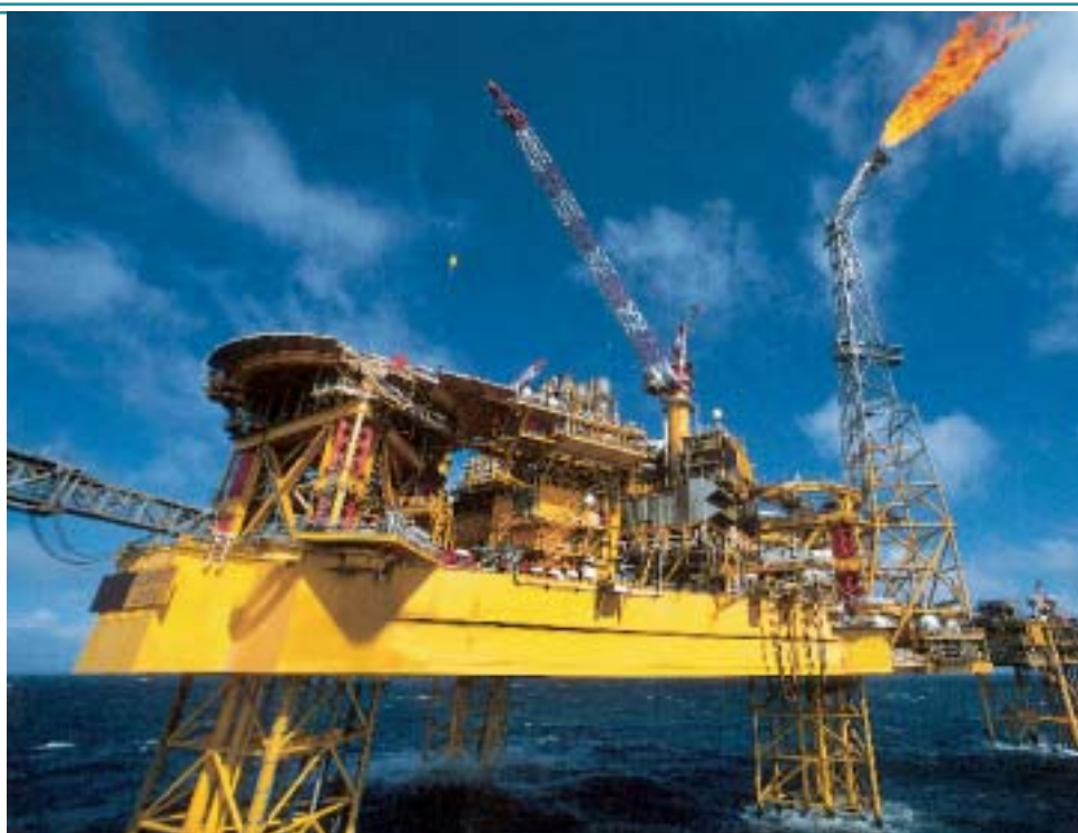
The PUQ jack-up platform, a mini oil and gas refinery with a sophisticated process system onboard to produce commercial quality gas.
