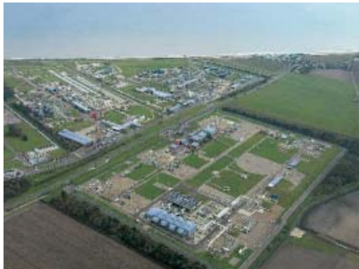
View of Bacton reception facilities from which gas is exported to the National Transmission System or to the Interconnector.
