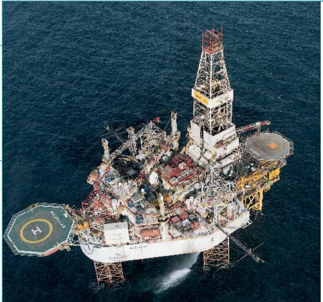
Aerial view of Global Santa Fe's Magellan drilling rig, working in cantilever mode to drill Franklin's production wells.
