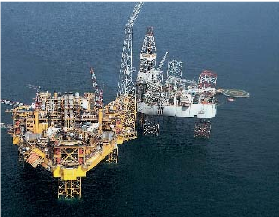
The PUQ and Elgin wellhead platform with the Galaxy-1 drilling rig and Polyconcord flotel alongside. Positively influenced by giving incentives to key contractors, the average drilling time per well was far better than expected.
