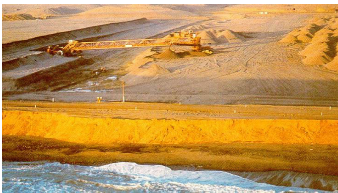
Figure 6: Example of beach diamond mining operations in Namibia
