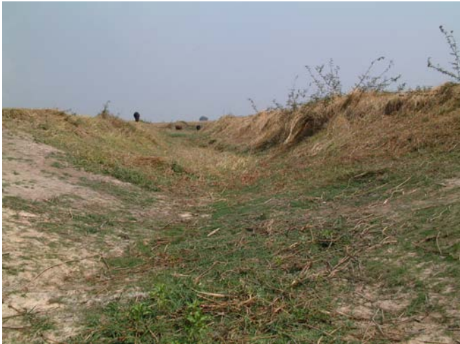
Figure 13: Example of hand-dug dyke, constructed originally at the start of the twentieth century, now fallen into disuse (Libonda district, Western Zambia, November 2003).
