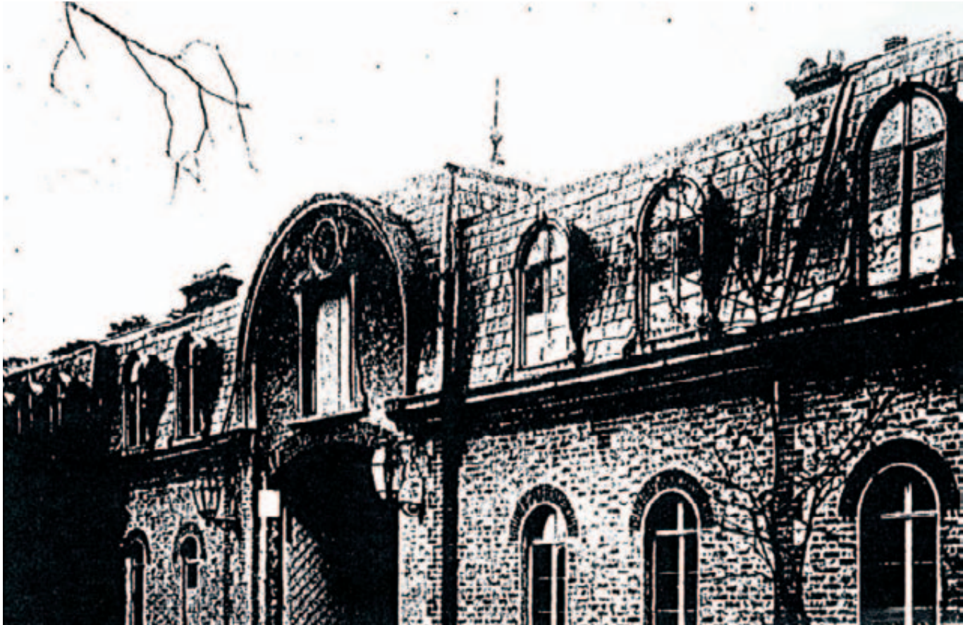
Orleans House Coach House, before removal of second storey photograph
