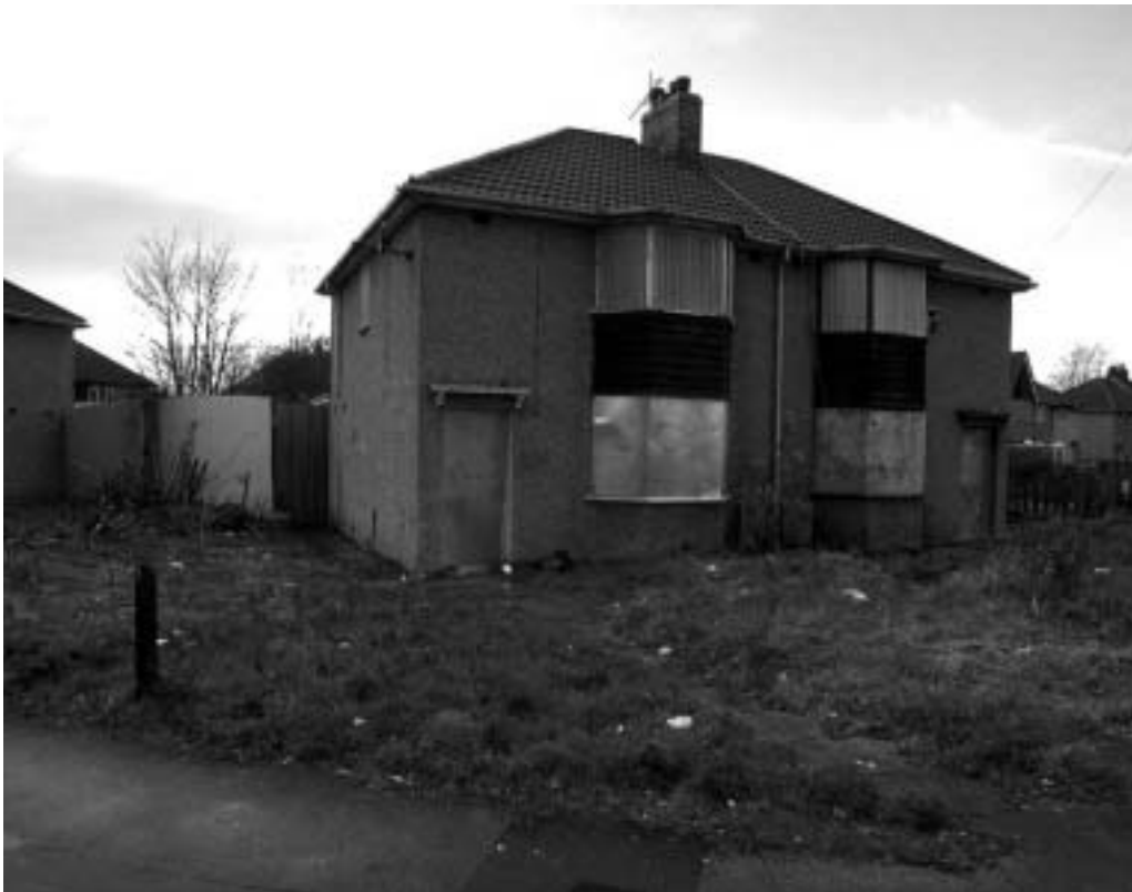
Photo 2: Norris Green, 1930s Boot estate earmarked for demolition
