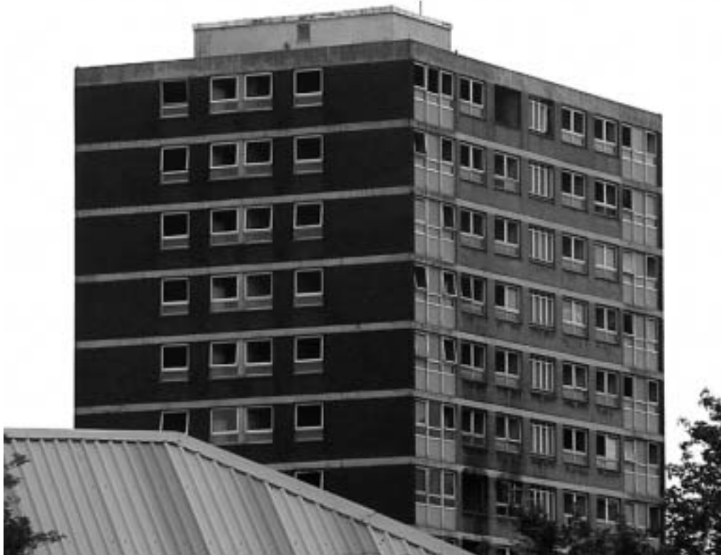
Photo 1: Ancoats, north-eastern Manchester; vacant tower block awaiting demolition
