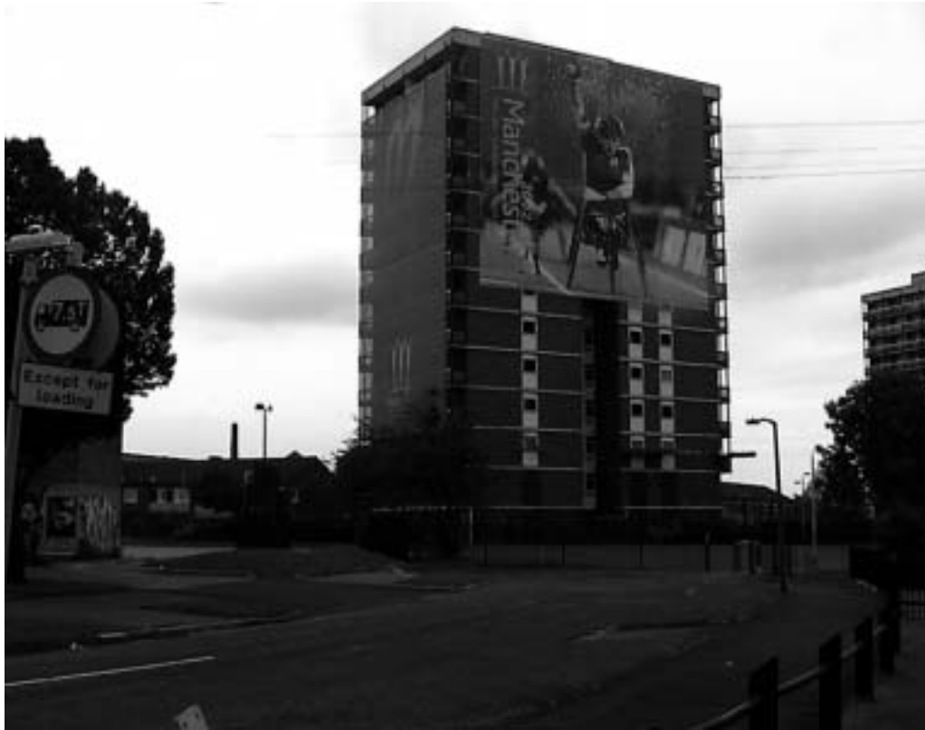
Photo 9: Billboard advertising the 2002 World Commonwealth Games attached to an Ancoats tower block, earmarked for demolition
