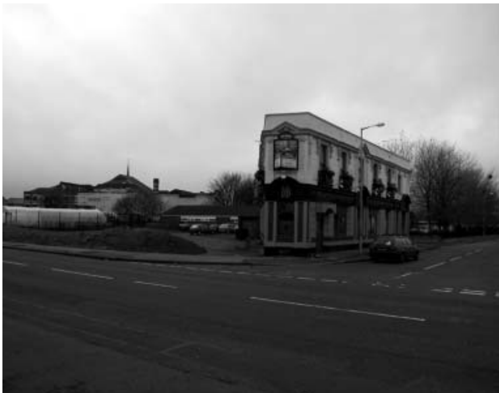
Photo 10: Hulme — 19th-century pub remains after tabula rasa demolition programme
