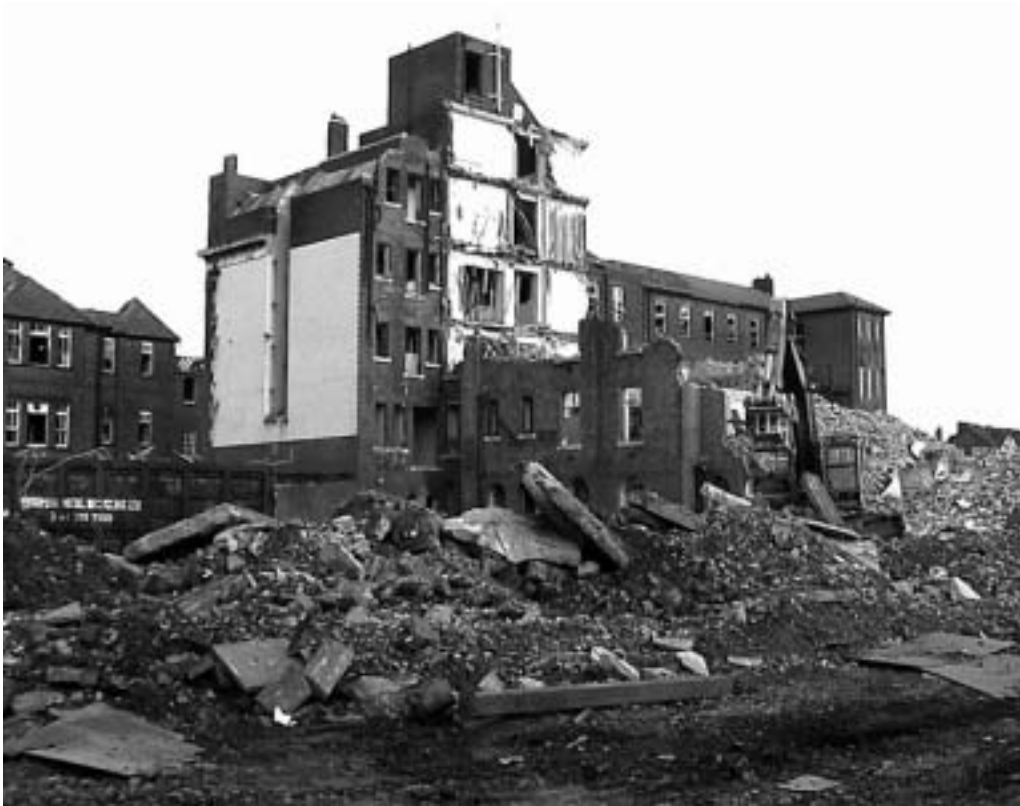
Photo 3: Rochadale Canal, Warehouses being demolished for redevelopment
