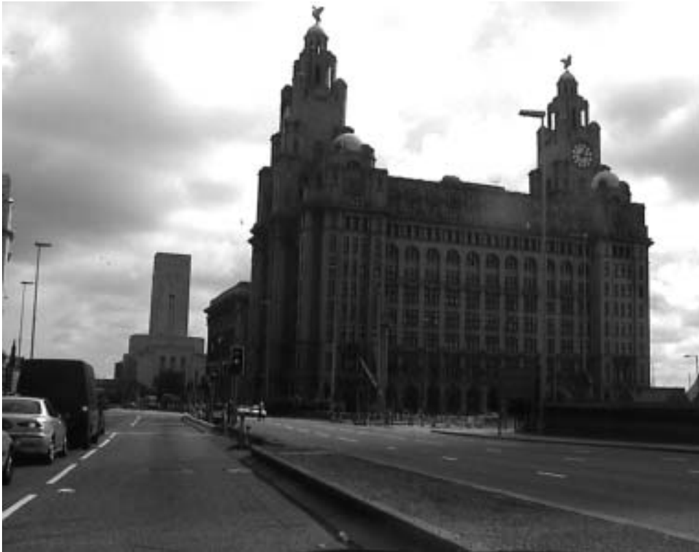
Photo 3: Liver Building, erected in 1910 as one of The Three Graces; one of the world's first multi-storey buildings with a reinforced concrete structure, marking the height of the city's power
