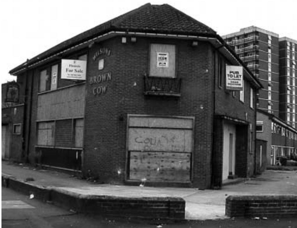
Photo 2: Disused pub — Cardroom Estate, East Manchester
