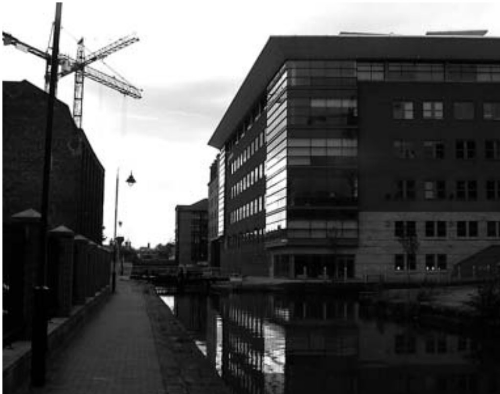
Photo 6: New office complex, Rochdale Canal area
