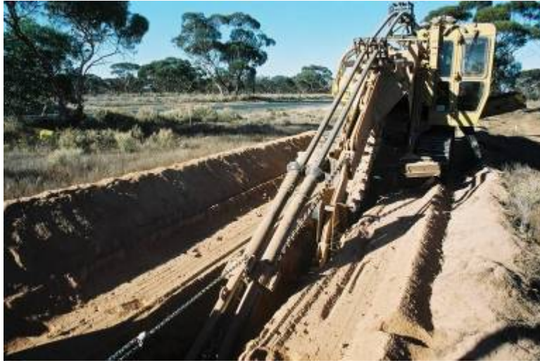
Fig 2. Cable laying in Australia
