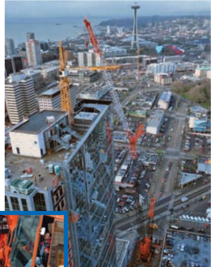
Local 302 Crane Operator and Executive Board Member Taylor Mayfield II, inset photo, is seen here operating a Manitowoc Maxer on the 8th West project in downtown Seattle for contractor Ness Cranes. The $3.2 million Maxer can lift up to 32,000 lbs. at a 160-foot radius.
