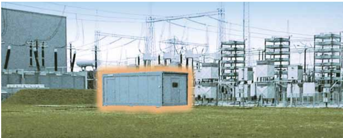
Fig. 5.4.3-5: Installation of the active AC filter, 400-kV substation Tjele (Denmark)
