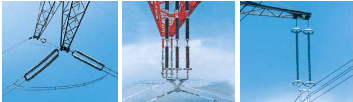
Example/Comparison of Insulator Application for a 400 kV Transmission Line
