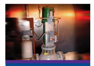
"We now have FIELDVUE DVCs on the toughest applications in this plant, including the valves controlling desuperheating spraywater, boiler feedwater, dearator inlets, and the soot blowers. They helped identify soot blower valve leaks that were losing as much as \$250,000 worth of steam per year. These losses were eliminated through a combination of corrective actions."
