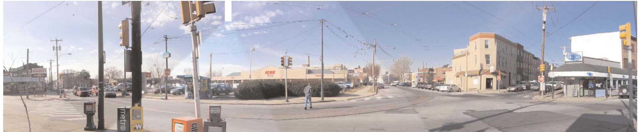
Because three major streets - Passyunk Avenue, Reed and 10th Streets- converge here in South Philadelphia, a vast paved surface results that accommodates vehicles, whether they be automobiles, trucks or buses. Pedestrians move through this intersection the best they can, often times ignoring established crossings.
