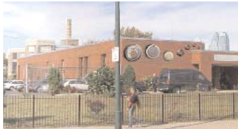
A blank building wall can be utilized for public art
