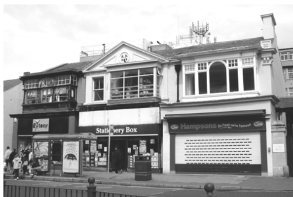
Plate 16: Shops on Abingdon Street, with inserted first floor bay windows, an indication of their use as lodging rooms
