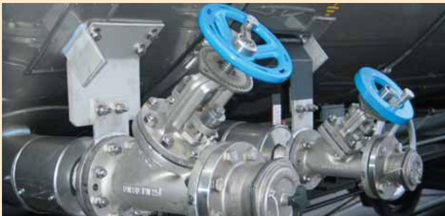
Figure 1: disconnect coupling, 80 mm for liquid line (left side), 50 mm for the vapour line
