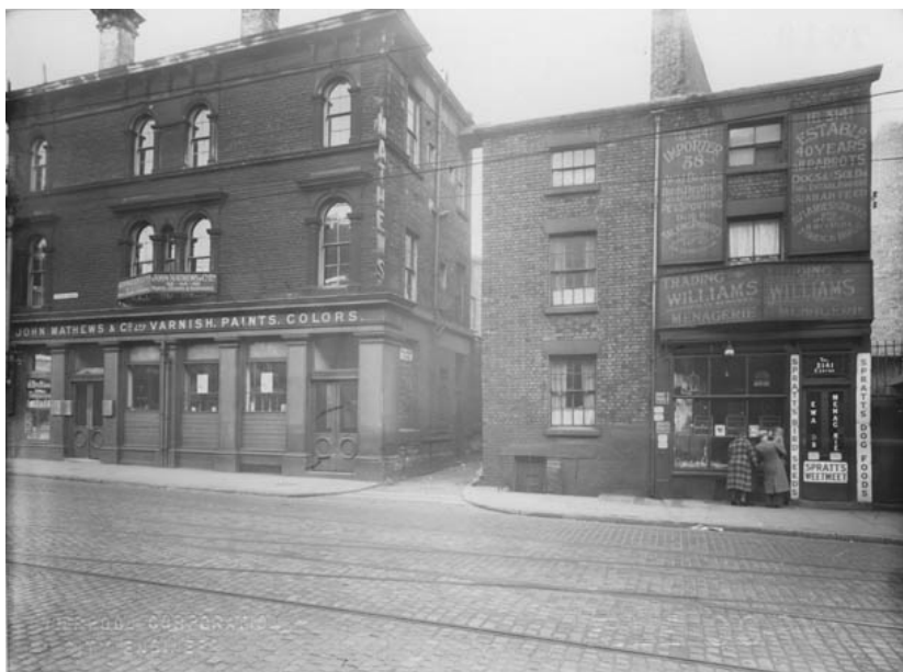
38 and 40 Hatton Garden to the right of Walkers Place
