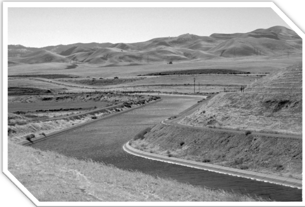
State Water Project – California Aqueduct
