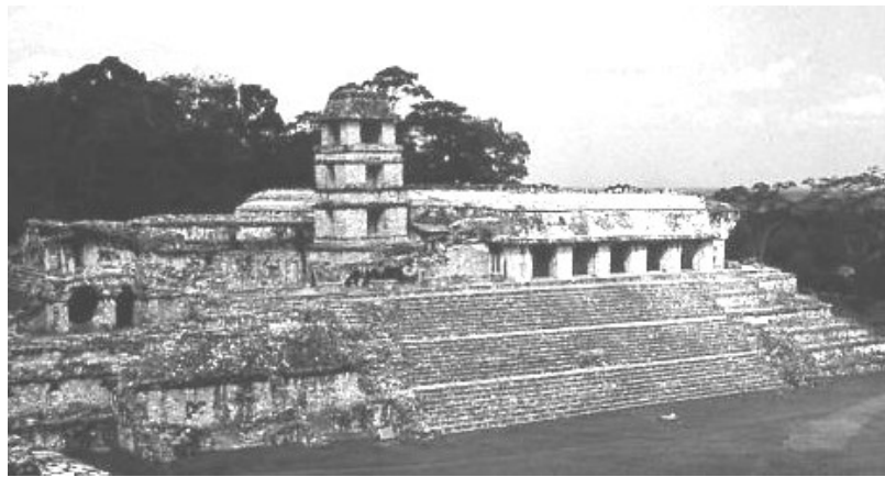
Figure 5.9 Narrow masonry piers on the Palace at Palenque, Chiapas.
