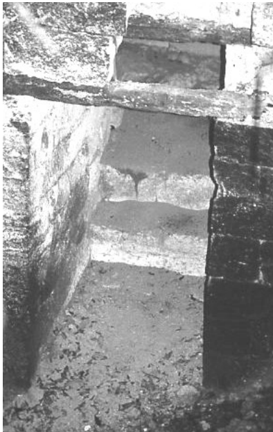
Figure 5.5 Chicozapote lintel in place at Manos Rojas, Campeche.
