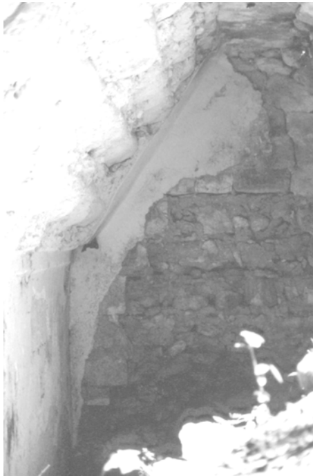
Figure 5.2 Note the difference in masonry between the side wall (in rear of picture) and the front wall in this structure at Manos Rojas, Campeche.
