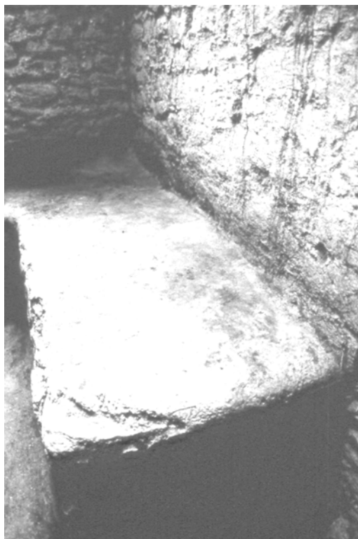
Figure 5.4 Note the lack of interlocking bond on the back corner of this structure (Structure EP22W in Plaza Jobo, El Pilar) and the difference in masonry technique between the two walls.
