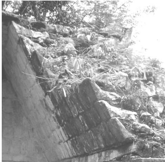
Figure 6.3 “Boot-shaped” vault stones in a vault at Chichen Itza, Yucatan.
