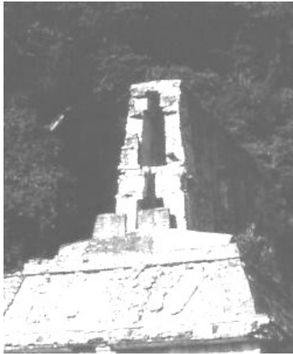
Figure 6.17 Side view of roof crest construction at Palenque, Chiapas
