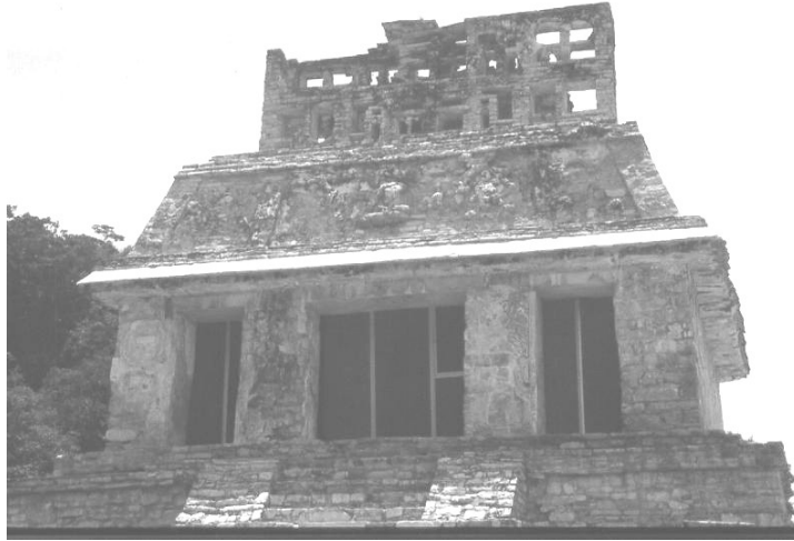
Figure 6.18 Front view of roof crest construction at Palenque, Chiapas.
