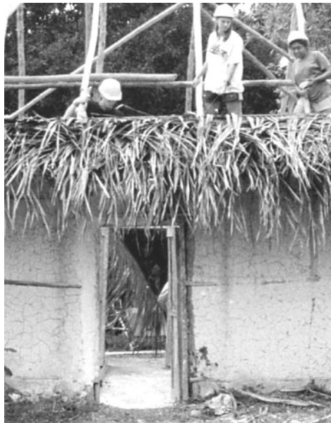
Figure 4.1 The sascab floor is visible through the door of this bajareque structure.
