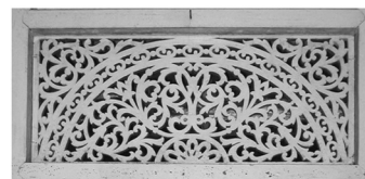
Ventilation panel of a palace door
