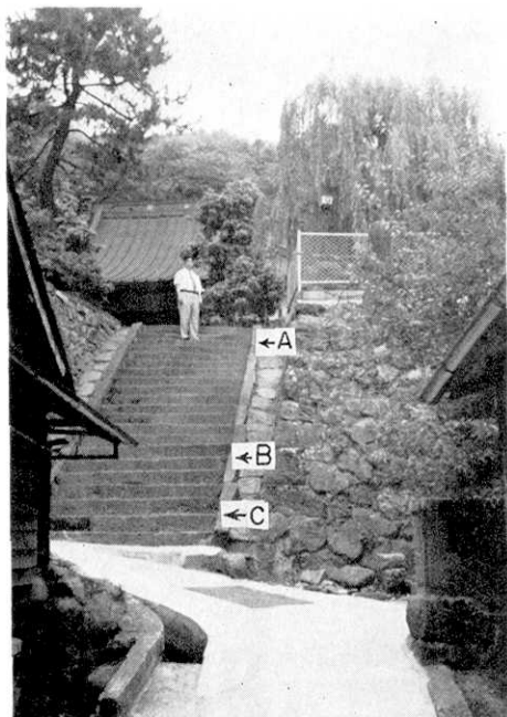
Fig. 4a. Inundation levels at the Kaizoji Temple in Kawana. A: the 1703 Genroku tsunami, B: the 1923 Kanto tsunami, C: the 1854 Ansei tsunami. The tsunami heights are 8.2m, 5.3m and 4.5 m above M. S. L.
