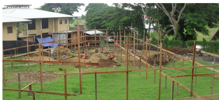
Profiling the Lecture theatre and digging of foundation has started.
