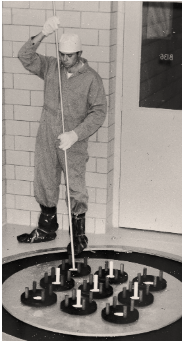
A mockup of the SL-1 reactor top. Analysts tried to determine where the three cadremen were standing at the moment of the accident.
