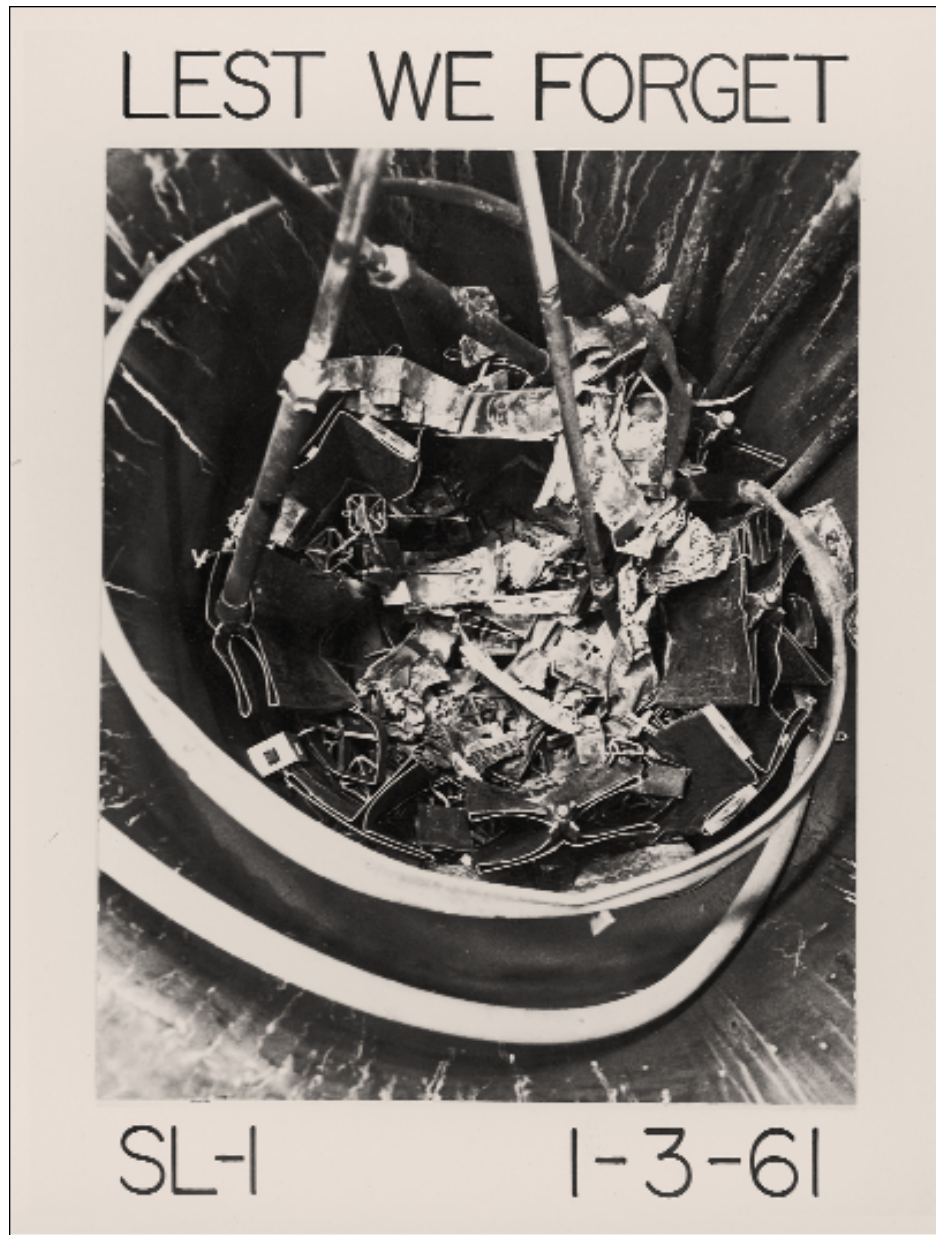
A 1961 photograph of the damaged top of the SL-1 reactor vessel was reused in 1981 to convey a safety message.
