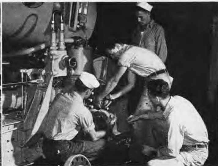
Training school students at NAF inspect cross-head sheave wheels on H4. Perfection of catapult boosted striking power of Navy flattops
