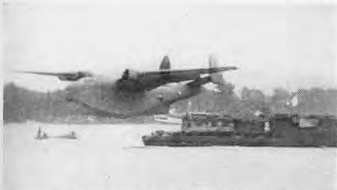
GIANT CATAPULT LAUNCHES A MARINER FROM ITS LENGTHY RUNWAY
