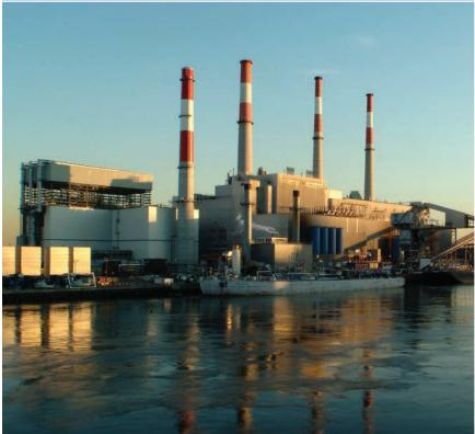
Ravenswood Generating Station (Ravenswood), located in Queens, NY, is a 2,480 megawatt (MW) power plant that consists of multiple units employing steam turbine, combined cycle and combustion turbine technology.
