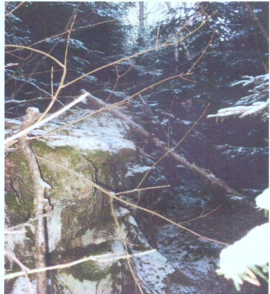
abandoned section: retaining wall for service road
