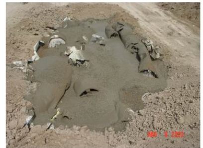
Pit filled with concrete 03
