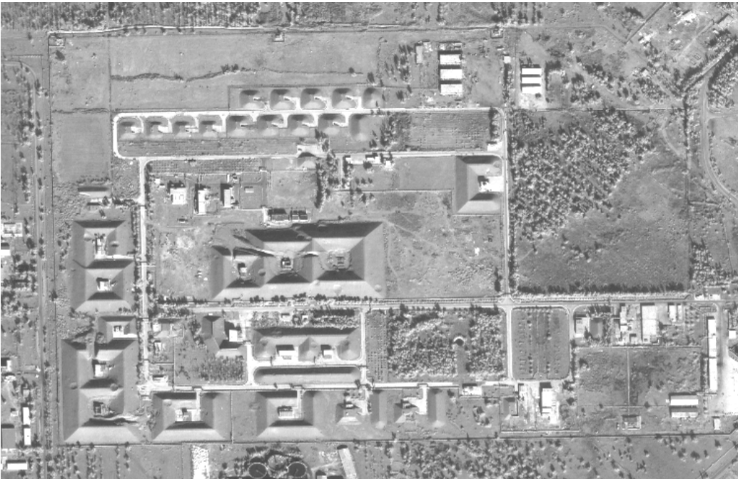
Figure IV.II.XVI Al Mamoun plant in November 1998
