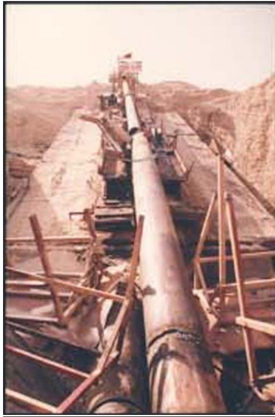
Figure IV.VII.IX Destruction of the 350mm diameter Supergun at Jebel Himreen site
