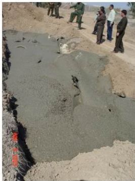
Pit filled with concrete 01
