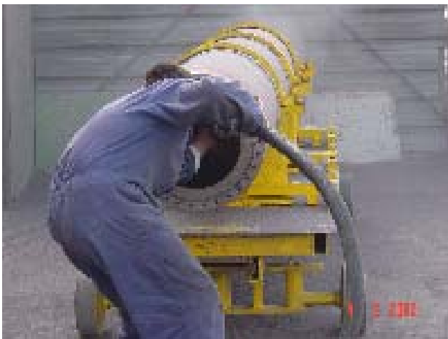
Figure IV.IX.XXXI - Grit blasting of motor case – Al Mamoun
