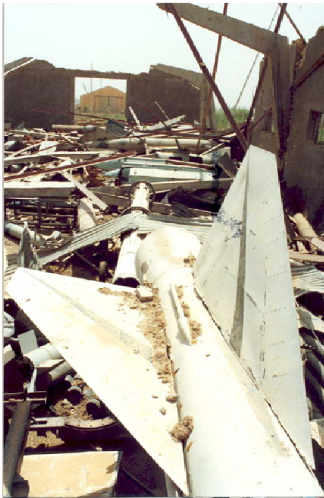
Figure IV.IV.II: Damaged Fahad 300 missiles in building destroyed in the 1991 Gulf War.
