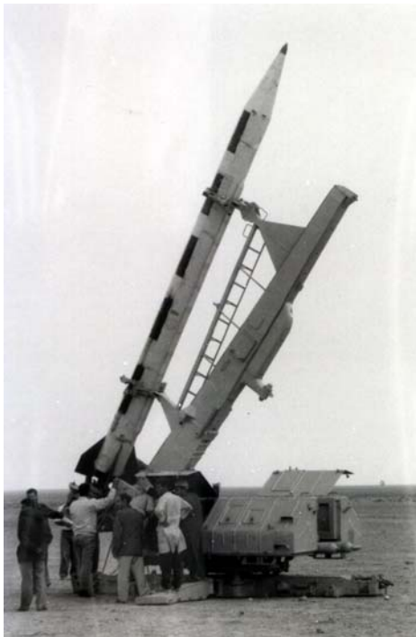
Figure IV.VIII.VIII - Al Samoud (500mm) on modified SA-2 launcher
