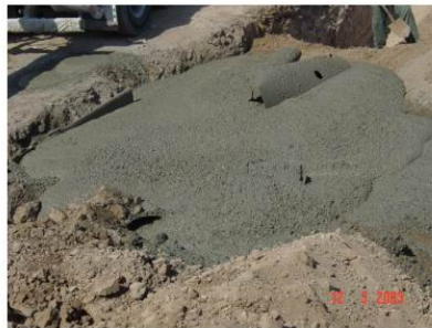
Pit filled with concrete 02
