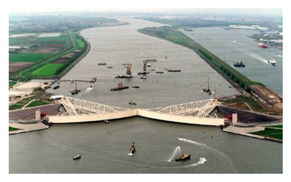
Figure 24. Stormvloedkering, sector gates which are rotated across the New Waterway in Holland, then sunk to provide the storm surge barrier.
