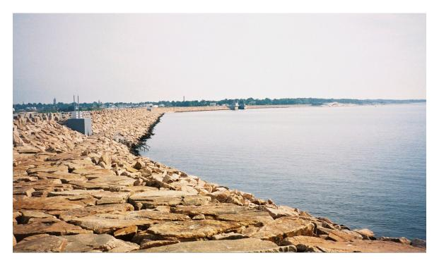
Figure 20. Hurricane barrier at New Bedford, Massachusetts, looking east toward Fairhaven, showing the open sector gates in the distance and a conduit gate in the foreground.
