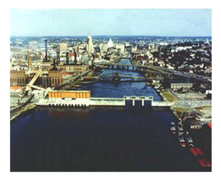
Figure 19. Hurricane barrier at Fox Point, Providence, Rhode Island, showing pump house on the left and three open tainter gates on the right.
