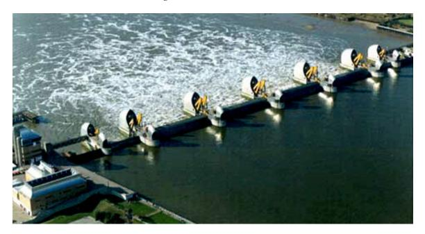
Figure 22. Thames River tidal barrier with the tainter gates in the undershot position, allowing the river current to scour out any accumulated sediment.
