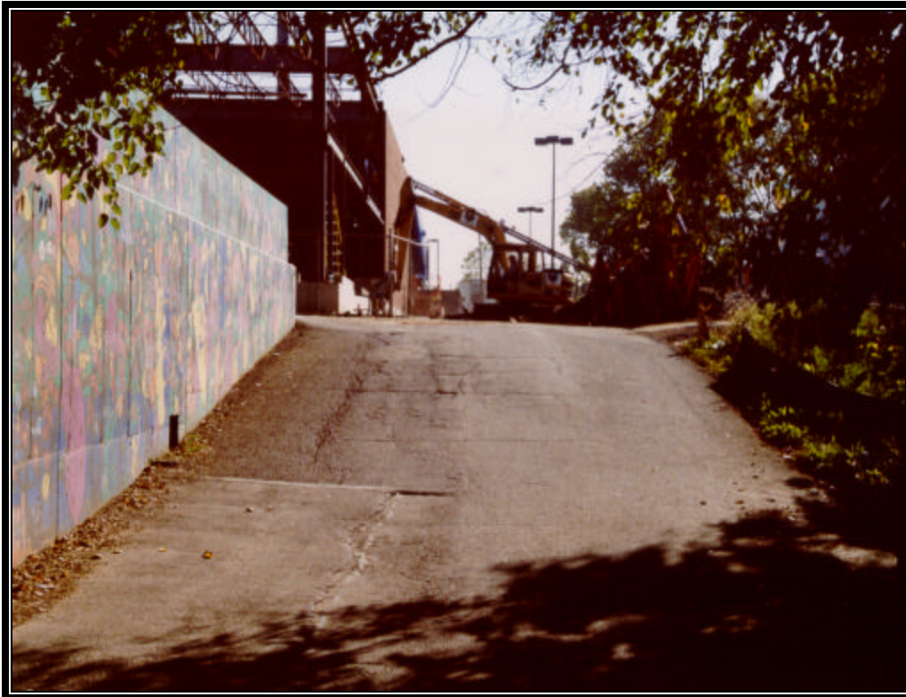
View of the Kroger access easement, another site of drainage problems
