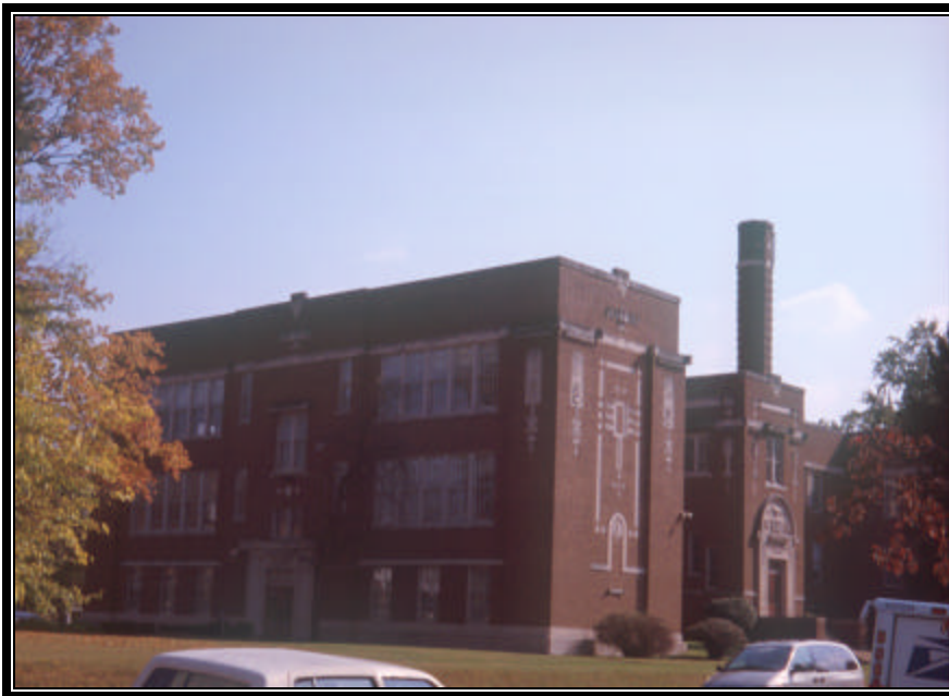
Belknap School – now converted to office uses.
