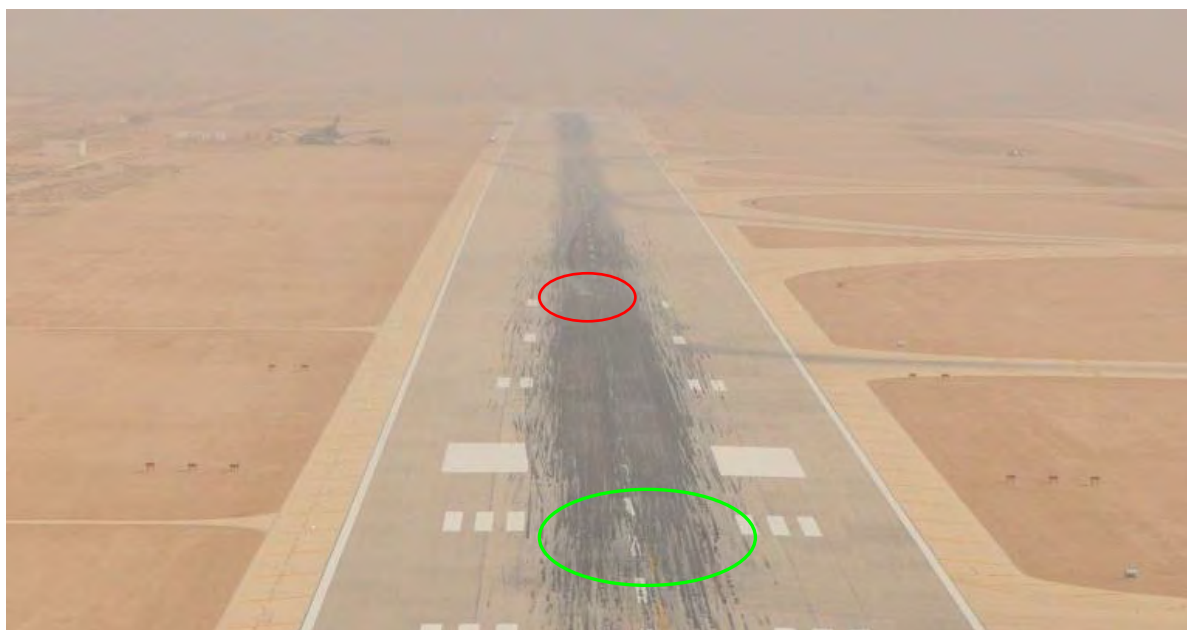
Figure 7: General View of Wreckage Trail
