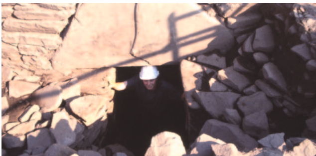
The broch lintel
