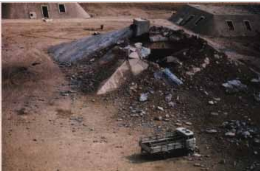
An Iraqi command bunker hit by a precision guided munition.
