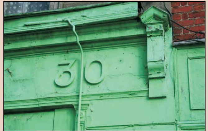
No. 30, Martin's Row, shop front detail
