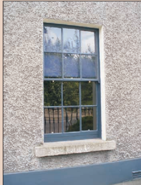
Timber sash window with early glass
