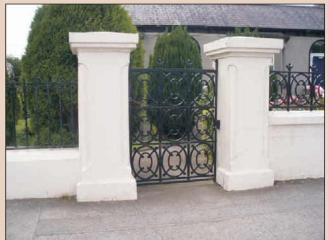
Cast-iron gate on Chapelizod Road
