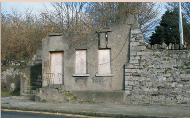
Derelict house, Gamble's Buildings, Main Street
