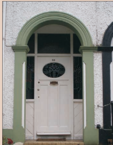
Timber panelled door in recessed porch
