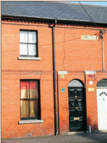
Brick-built dwelling, Liffey Terrace
