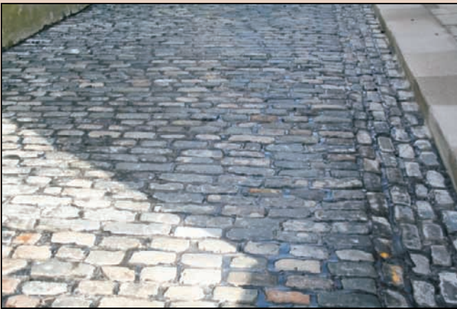
Recently refurbished sett-work to Chapel Lane
