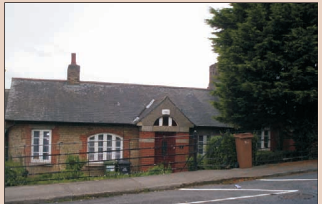
Chapelizod Hill cottage
