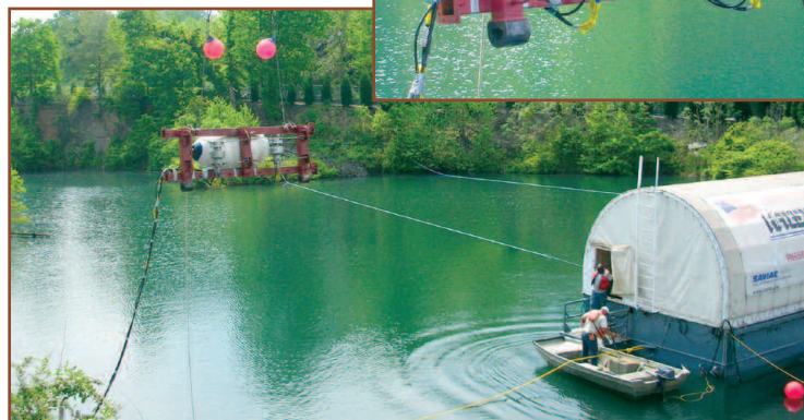
Below A framework with two air gun assemblies being lifted into place for testing.
