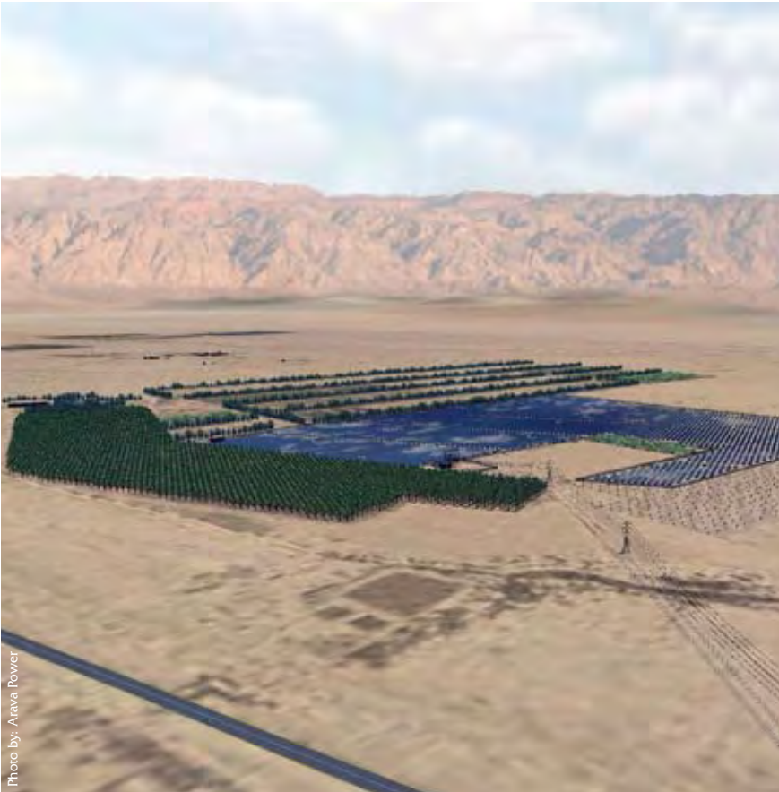
The 40 MW solar field to be built by Arava Power at Kibbutz Ketura will supply one-third of Eilat's energy needs during peak usage and eliminate the need for diesel generators.
