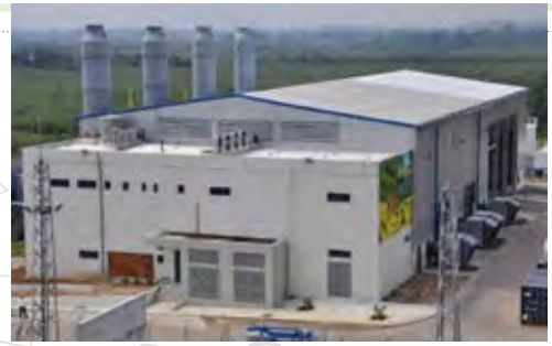
Gabon 70MW gas based power plant.
