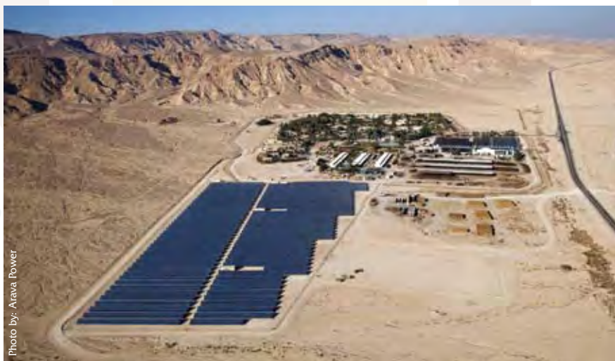
Arava Power's 4.95 MW solar field has been operational for over a year with production levels that exceeded the company's expectations.
