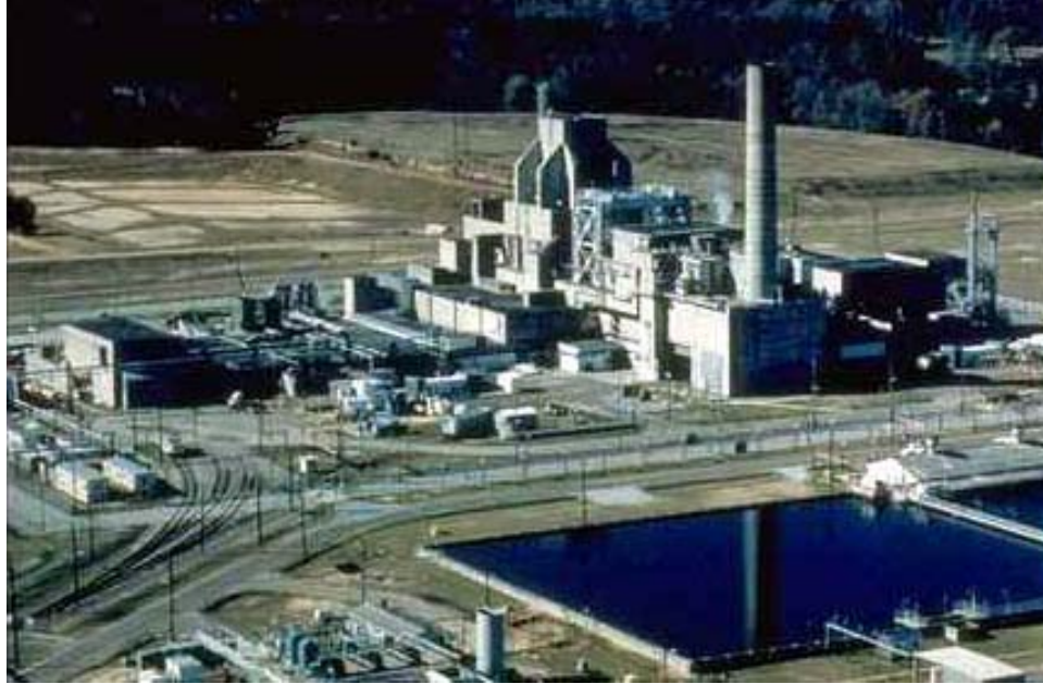
Fig. 13: Savannah River Heavy Water Reactor for the production of tritium from highly enriched U^{235} naval reactors fuel in LiAl alloy.
