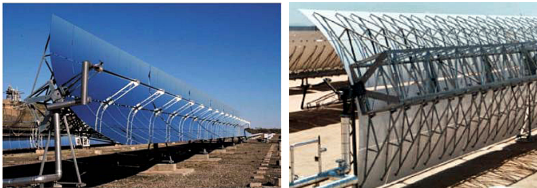
Figure 29. Front and back views of parabolic trough Skal-Et 150 at Al Kuraymat, Egypt, 2010. Peak optical efficiency: 80 percent. Geometric concentration: 82. Length: 123.75 m / SCA. Aperture area: 817.5 \text{ m}^2/\text{SCA} [16].
