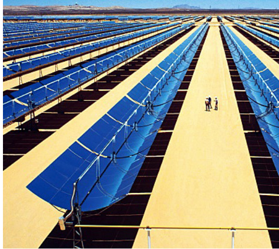
Figure 35. Kramer Junction solar plant, USA.
