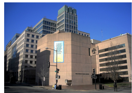
The proposed demolition of the Third Church of Christ, Scientist in Washington, D.C. has resulted in court battles between historic preservationists and church members.
