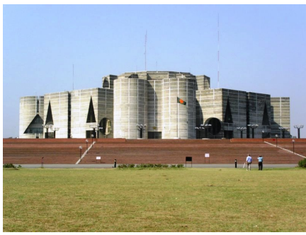
The Jatiyo Sangshad Bhaban (National Assembly Building of Bangladesh), 1961-1981, by Louis Kahn.
