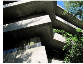
The John Andrews Building of the University of Toronto Scarborough
