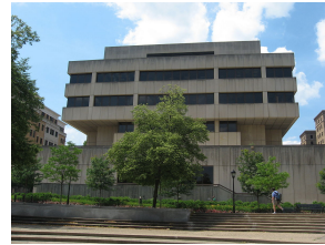
The Barco Law Building at the University of Pittsburgh School of Law
