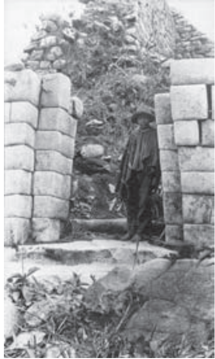
Fig. 11 Photograph of the double-jamb entryway to an elite household (the Ingenuity Group) at Machu Picchu taken by Hiram Bingham III. Courtesy of the Peabody Museum of Natural History, Yale University.
