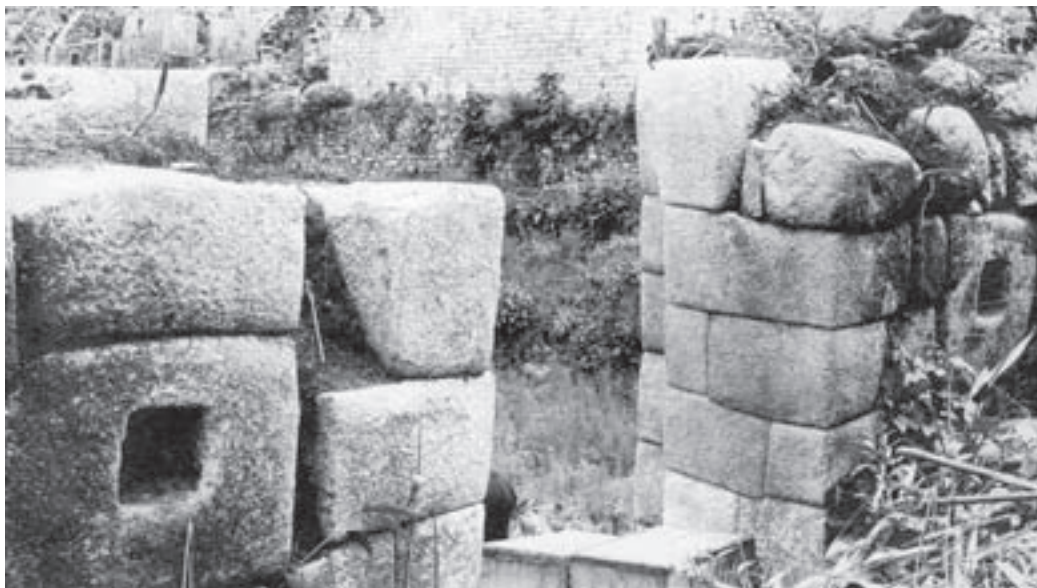
Fig. 13 Bar-holds used to block entrance to the elite compound known as the Ingenuity Group. Photograph by Hiram Bingham III, courtesy of the Peabody Museum of Natural History, Yale University.
