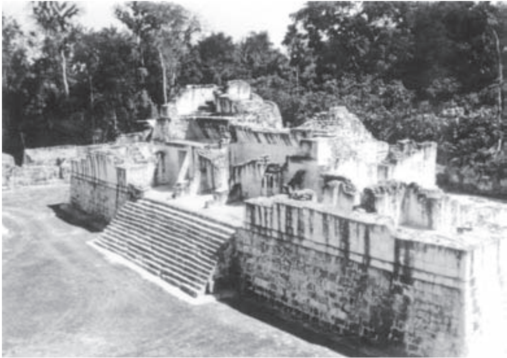
Fig. 5 Structure 5D-46, after excavation and partial reconstruction. Its central core is the Early Classic house of Jaguar Claw the Great (Chak Toh Ich'aak), which was built in the mid-fourth century. An inscribed cache vessel (see Fig. 6) was recovered beneath the west stair.
