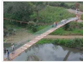
Puente Quebrado Veracruz, Mexico 12.02.2003 71.83m
