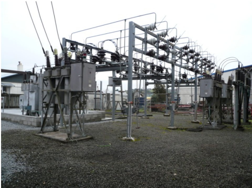
Figure 6-19 : Swanson before redevelopment
