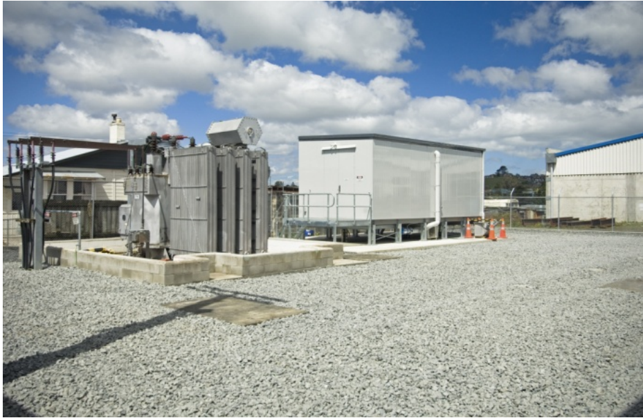
Figure 6-20 : Swanson after redevelopment
