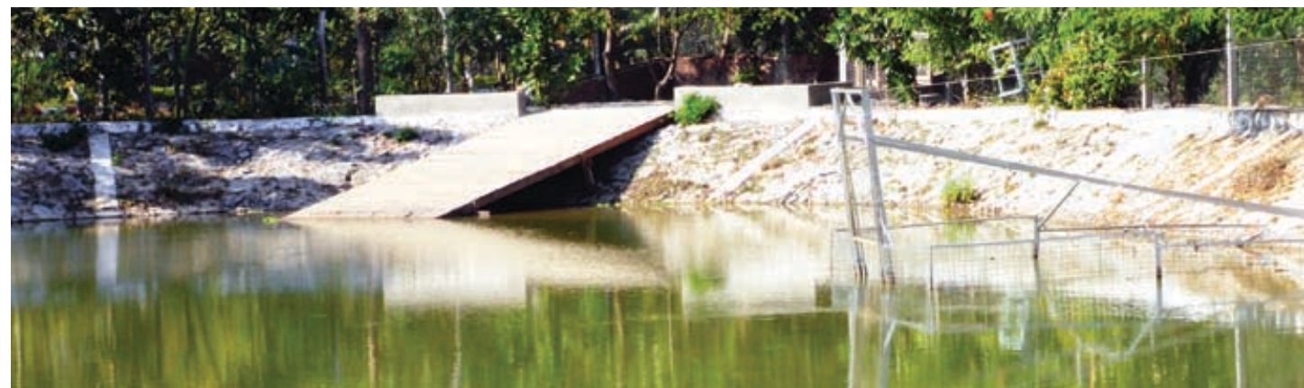
The new breeding pond at the Yadanabon Zoo is large and features a nesting beach, a floating basking platform and a fenced feeding area to assist with capture.
