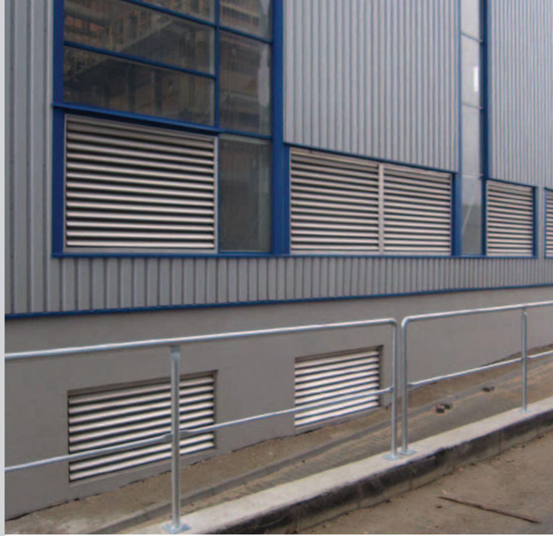
Colt Poland Stolze, Częstochowa Colt products: Attenuated Labyrinth natural ventilators and FCO ventilators
