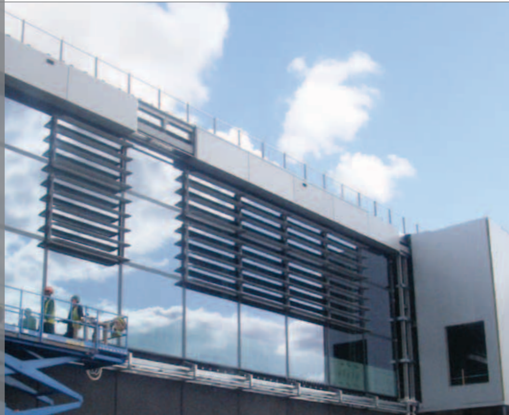
Colt UK Terminal 2, Heathrow Airport Colt products: Bespoke solar shading louvres and Universal Louvre
