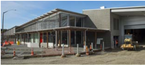
Newlands New World under construction
