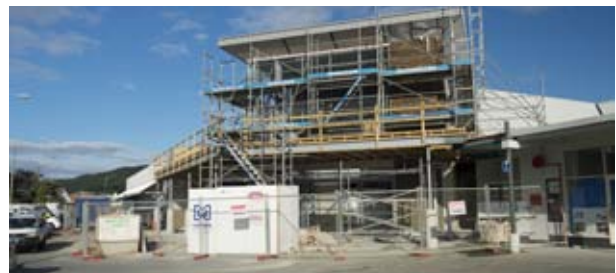
Tawa New World under construction
