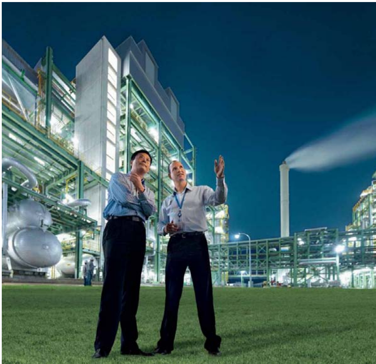
Construction of the Shanghai Chemical Industry Park in China requires close collaboration among international teams. The picture shows Bayer colleagues Dr. Yun Chen (left) from China and Dr. Mark Land from the U.S. in front of the new TDI facility.
