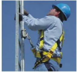
While the poles of both of these units appear similar, they are brand specific and not interchangeable. The only way to tell the two apart is by measuring the spacing between mounting bolts (on the back side of the rail); North mounting holes are spaced 9" apart, while the Antenna are nearly 10" apart. Ships that have the North product must use a Y lanyard when going aloft or replace North poles with the Antenna poles to utilize the ladder climbing device.
