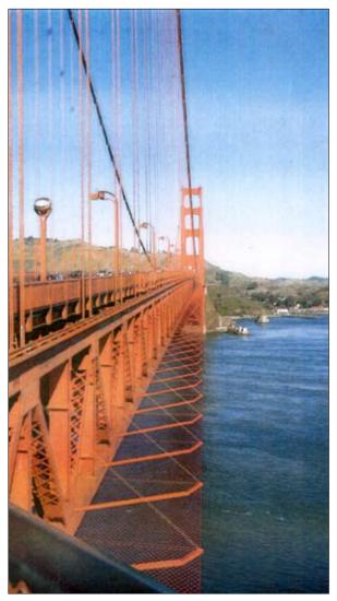
Photo simulation of the proposed net barrier designed by Caltrans to deter suicide attempts from the Golden Gate Bridge.
