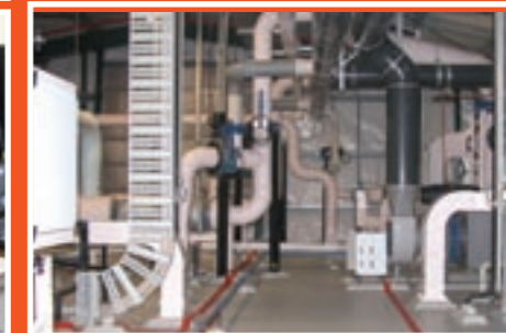
Below right: Part of the sophisticated airflow and filtering system that ensures any disease organism remains well and truly contained at the high-security PC3+ laboratory.
