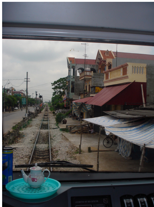
Photo 5. Occupied buildings are perilously close to the rails
