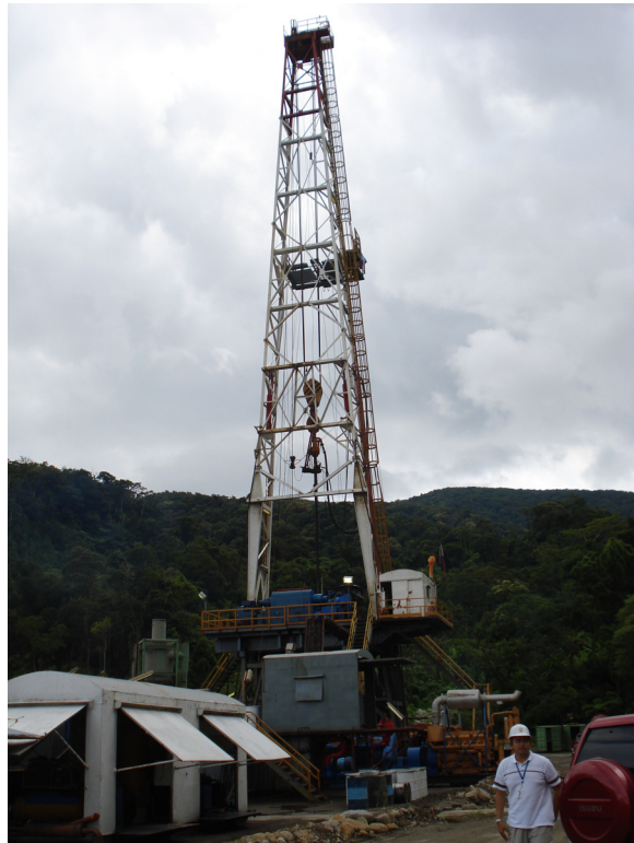
Photo 3. Drilling of new production well for topping off steam power
