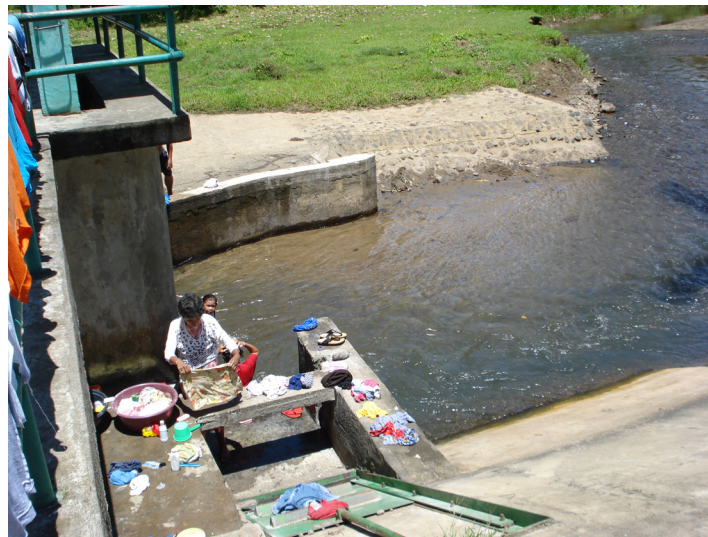
Photo 1. CIP ARISP Dam
