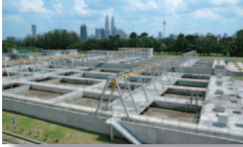
Sewage Treatment Plant in Malaysia built by Hitachi Plant Technologies
