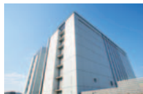
Data Center (Yokohama No. 3 Center)
