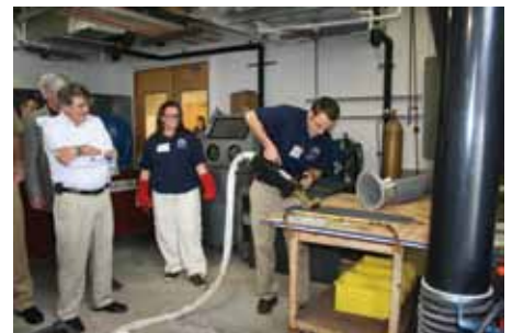
Demonstration of the removal of non-skid coating by heat induction at NRL Key West.
