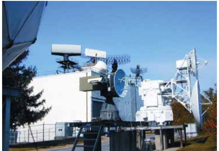
Radar antennas in front of and on the roof of the Radar Test Facility.
