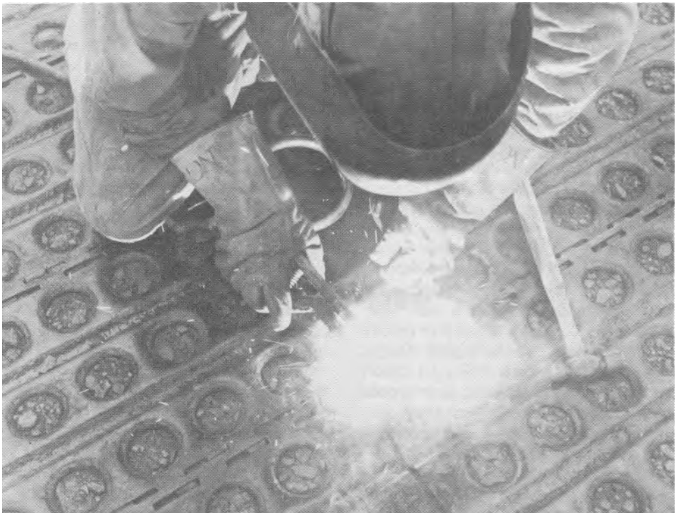
Locking slots and bayonet hooks are secured and welded by crews of the 930th Engineer Aviation Group of the U.S. Army.
