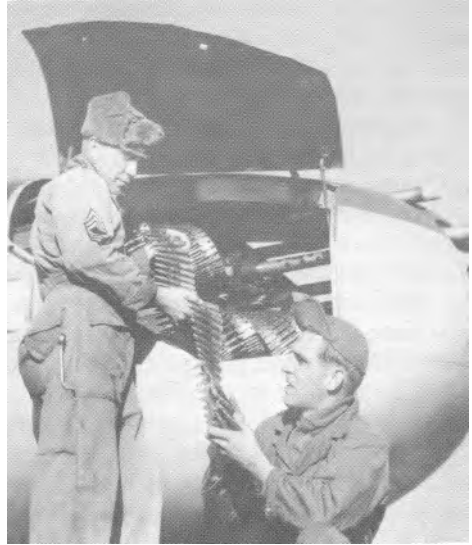
Loading .50-caliber machinegun rounds which will feed the nose, wing, and turret guns of the B-26.
