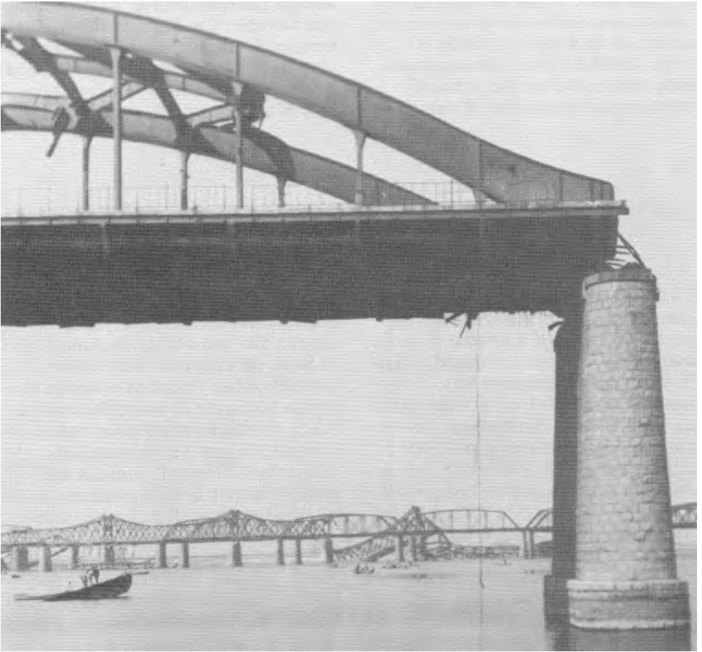
Bridge-busting activities on the Han River.
