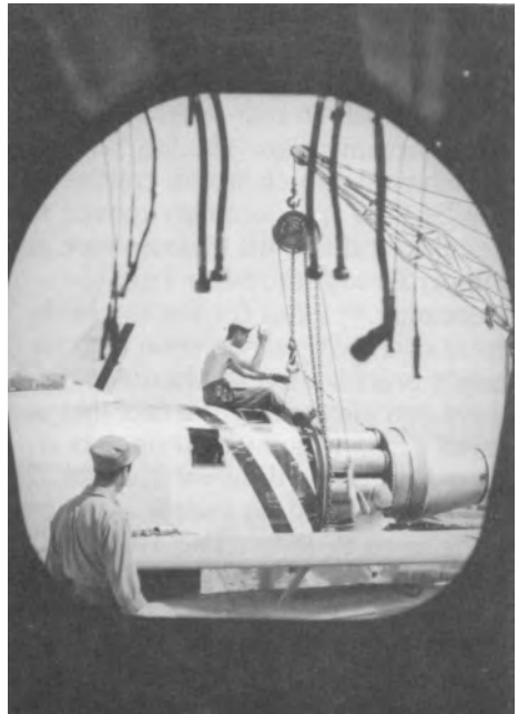
An aircraft maintenance crew hoists a Sabrejet engine into position for installation.
