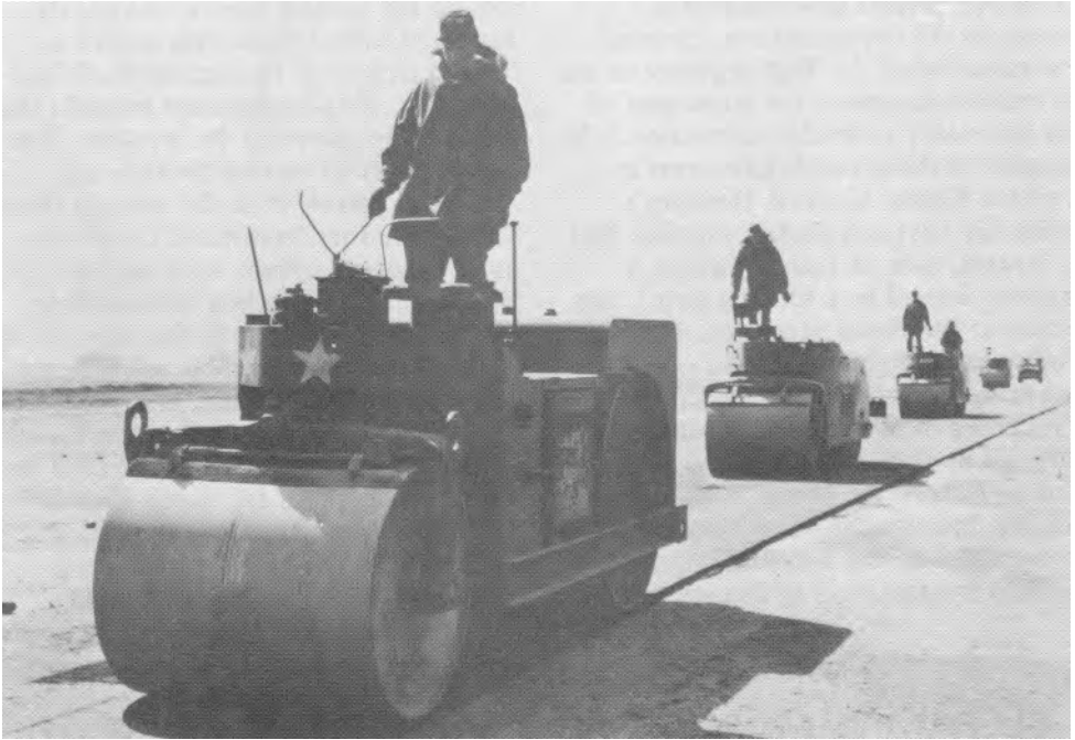
Rollers pack down the asphalt surface of a runway.
