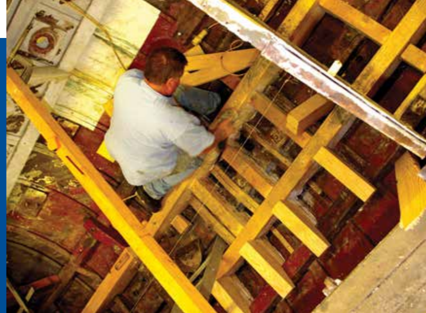
Replacement main engine mounts in place. Shipwright Steve is making precise adjustments to maintain correct shaft alignment.
