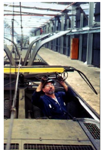
Replacing a Tangara pantograph at the Mortdale Maintenance Centre.
