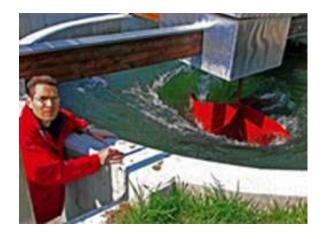
Austrian engineer, Franz Zotlöterer, has constructed a low-head power plant that makes use of the kinetic energy inherent in an artificially induced vortex. The plant can be installed with a water drop as little as 0.7 meters.
